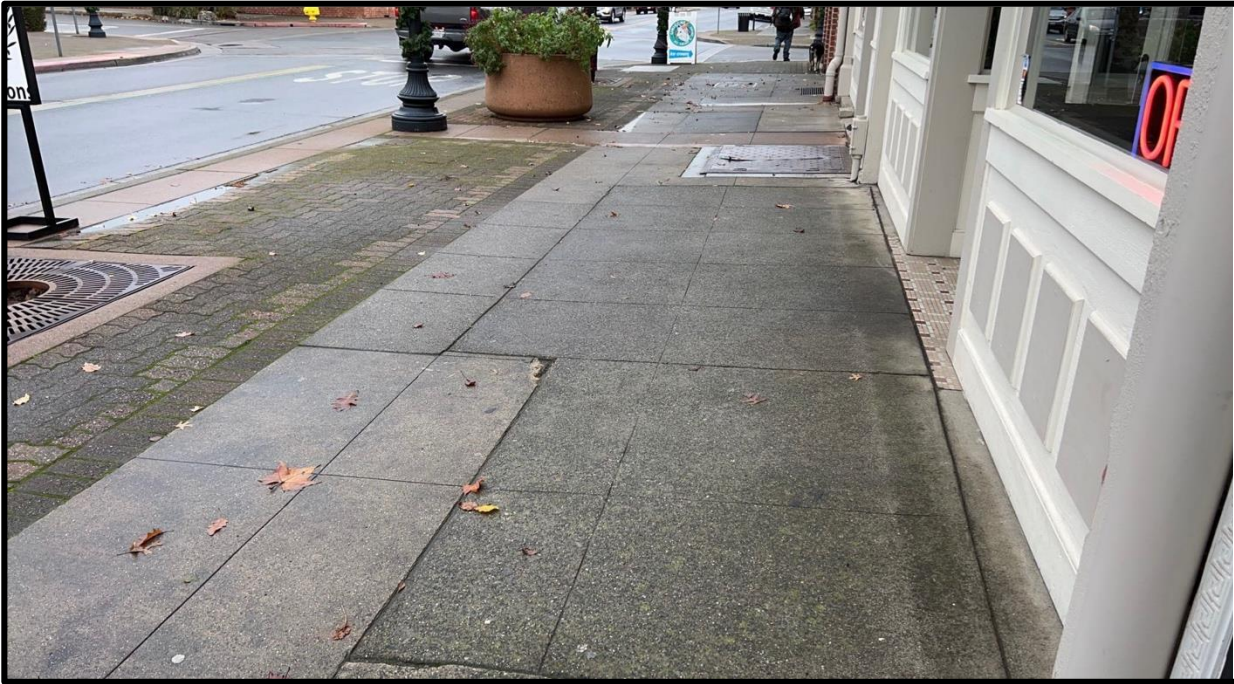
Figure 1: Existing Sidewalk on Montgomery Street
